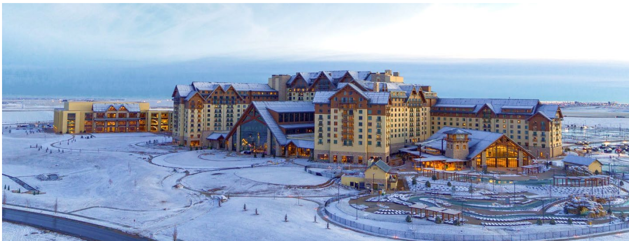
Figure 15. Gaylord Rockies. From Ryman Hospitality Properties. https://www.rymanhp.com/property/gaylord-rockies/ .
